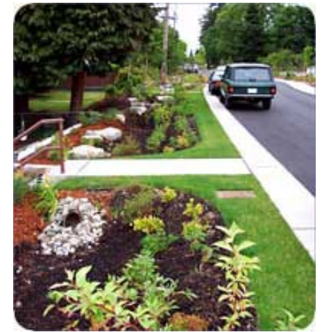
Bioswale along a Residential Street
