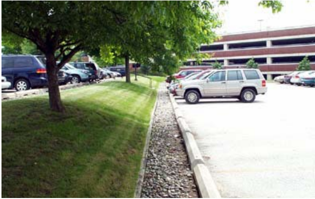
Infiltration beds in a parking lot
