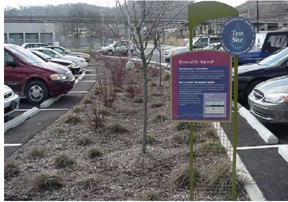
Bioretention swale in a parking area
