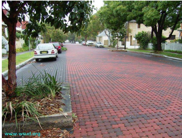
Permeable paver retro-fit for a residential street
