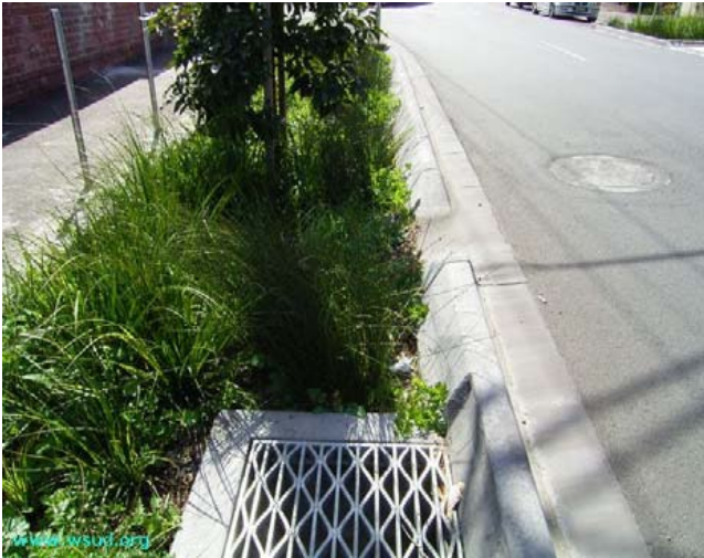
Bioretention swale retro-fit to roadway
