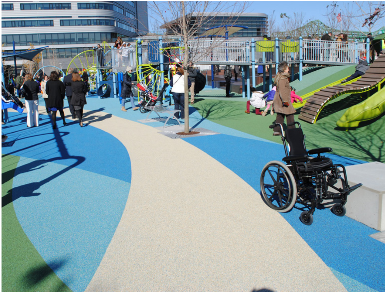
POURED-IN-PLACE SAFETY SURFACE
